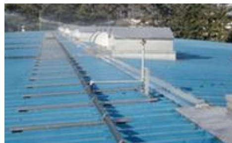
Running status of circulating roof spray system
